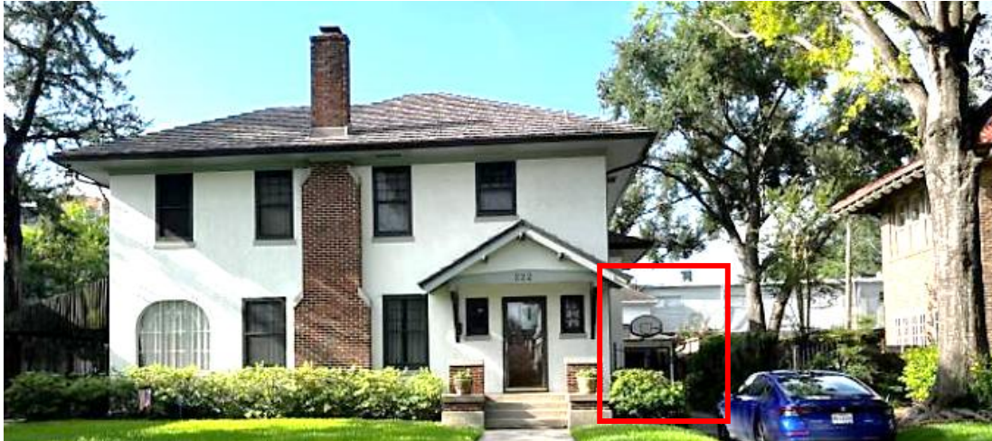
View of Existing Contributing section of Garage from Street
