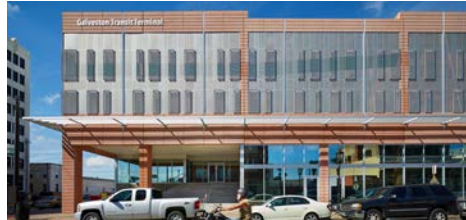
Galveston, TX – Downtown Transit Terminal – Innovative Development
