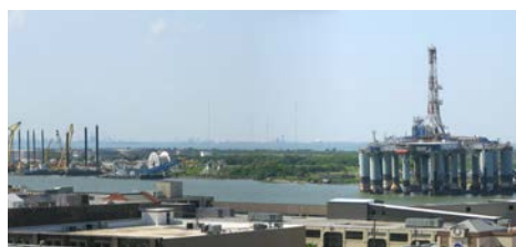
Galveston County, TX – Pelican Island Bridge Replacement
